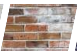
Efflorescence on Wall
